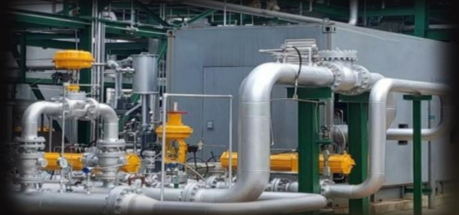
Energy Recovery Expansion Unit
