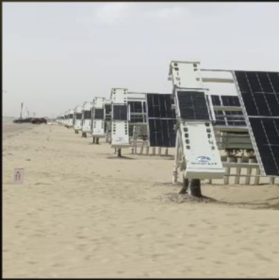
Large amount of dust working site
