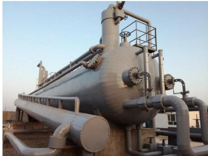
Our integrated water separation unit.
