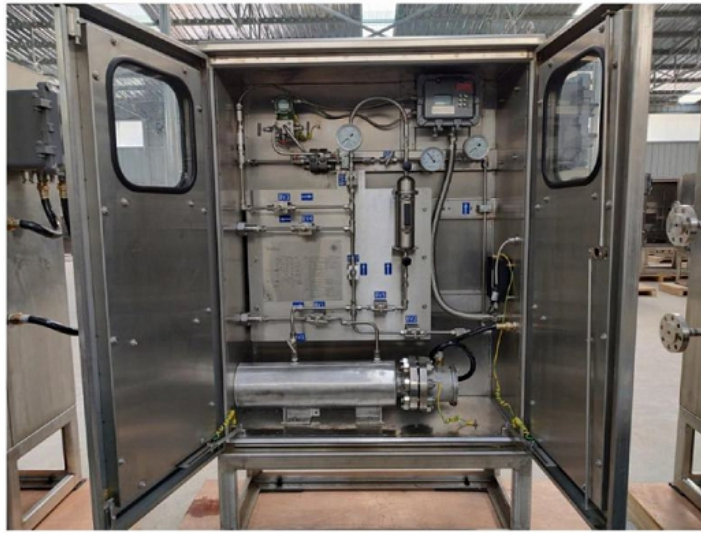
Our natural gas online sampling and analysis system.
