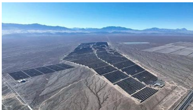
Yumen Oilfield Photovoltaic Project.
