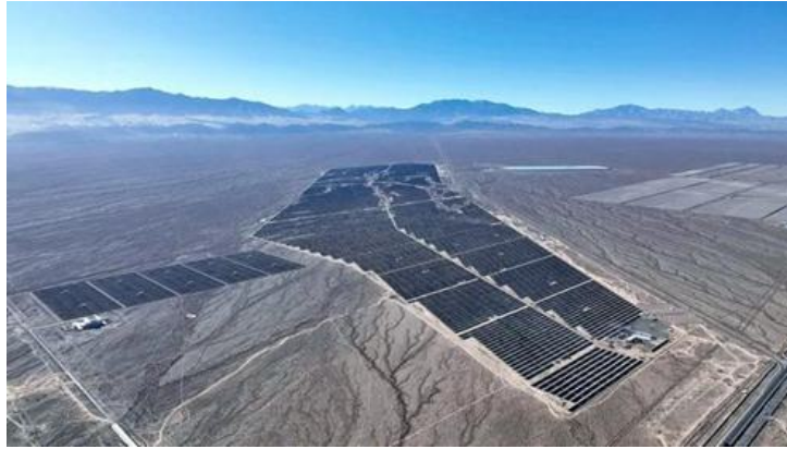
Yumen Oilfield Photovoltaic Project.
