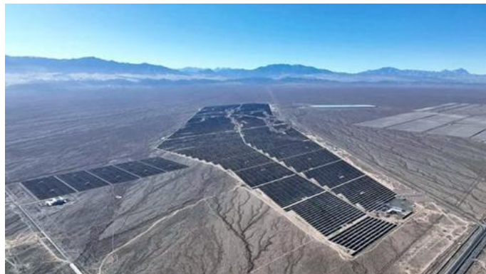
Yumen Oilfield Photovoltaic Project.
