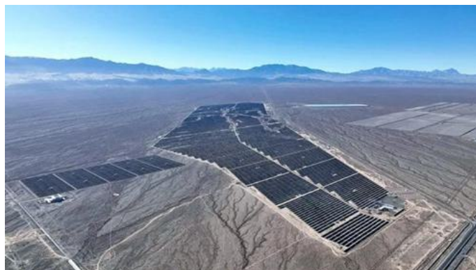
Yumen Oilfield Photovoltaic Project.
